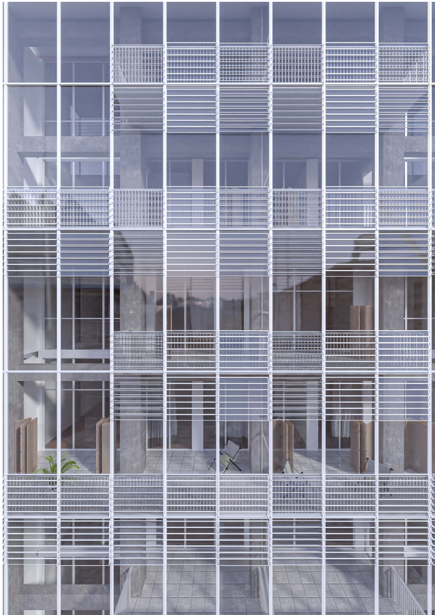
South facade renovation with wintergarden extension, creating a climatic buffer zone
